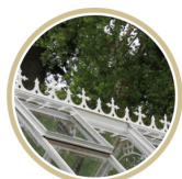
Cresting and finials
