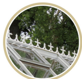
Cresting and finials
