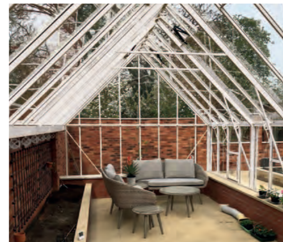
Valley gutter assembly interior with supporting Victorian style brackets
