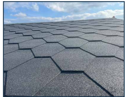
Roof is covered with heavy duty bitumen felt tiles as standard available in different colours
