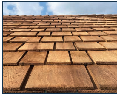
Optional Canadian Western Red cedar shingles fixed to pressure treated joists to enhance the appearance of your building and provide added protection to the roofing felt
