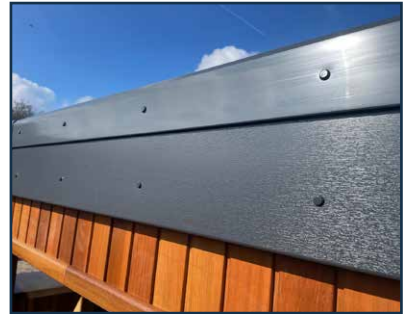
EPDM maintenance free synthetic one piece rubber membrane covering the roof with uPVC fascias and trims providing a maintenance-free finish to our roofs
