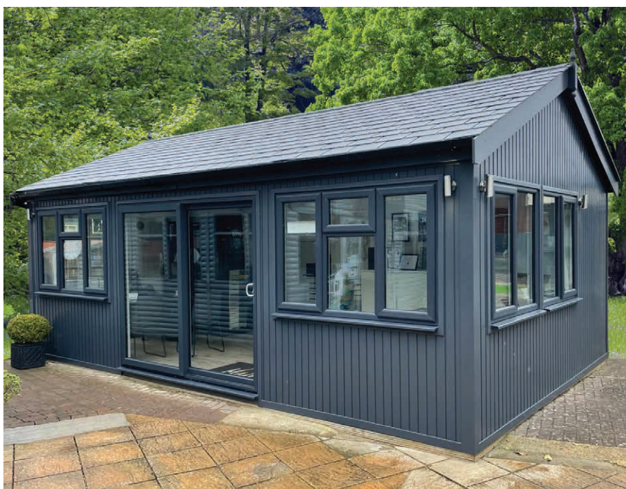
23' x 14' Hallow with uPVC casement windows and single sliding door
