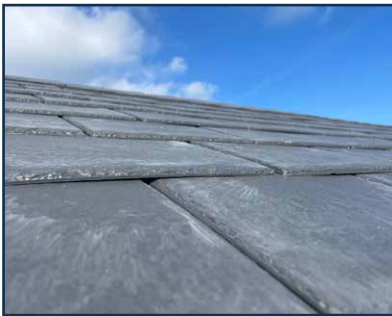
Optional slate effect tile is a synthetic roof tile which emulates the appearance of natural slate and has a long life span with no maintenance
